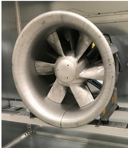
ZerAx® axial flow fan in AHU section
