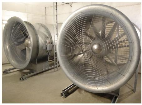
New high efficiency ZerAx® axial flow fans installed at Sima Power Station
